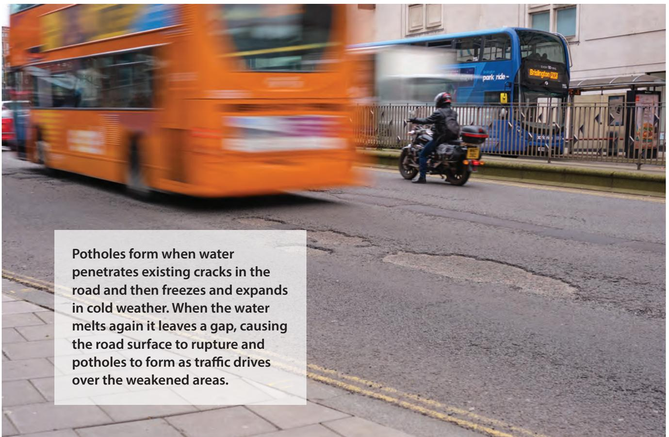
Potholes form when water penetrates existing cracks in the road and then freezes and expands in cold weather. When the water melts again it leaves a gap, causing the road surface to rupture and potholes to form as traffic drives over the weakened areas.
